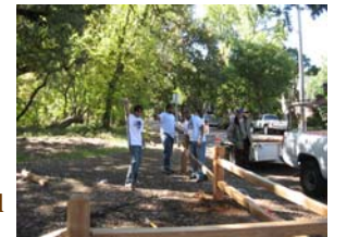
CSU students install split rail fence at One Mile.
