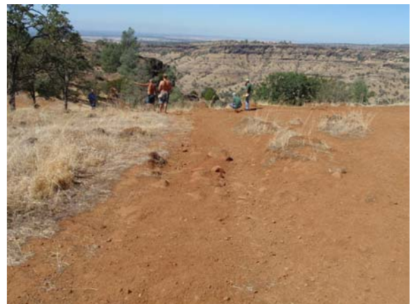
Photo 4: Path is eroding. More exposed rocks and less soil.
