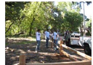
CSU students install split rail fence at One Mile.
