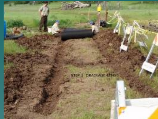
Drainage lens construction
