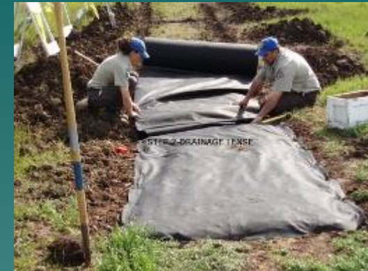
Drainage lens construction
