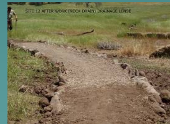
Finished drainage lens that allows water to pass under the trail.
