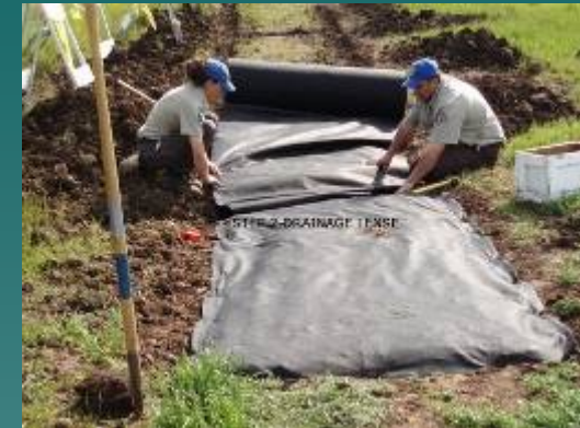
Drainage lens construction
